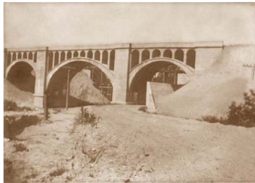
Bridge while under construction
