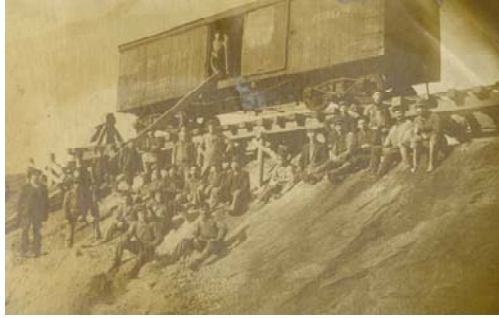
Workers shown preparing railroad trestle for bridge construction
