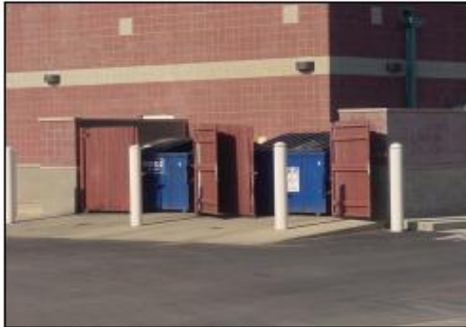
Figure 15: Screened Refuse Area
