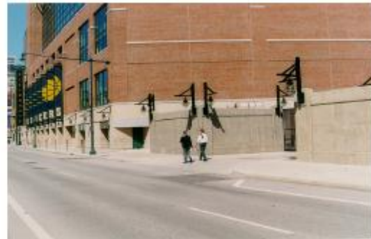
Figure 18: Example Loading Area
